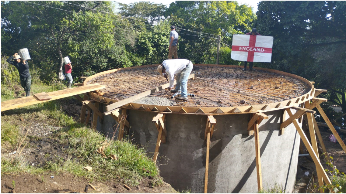
- FIRST YARULA TANK NEARING COMPLETION -
