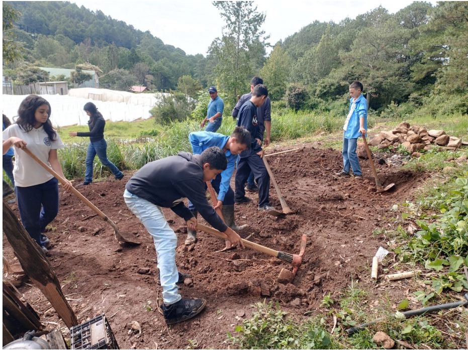
- PREPARING THE LAND FOR THE WATER TANK -
